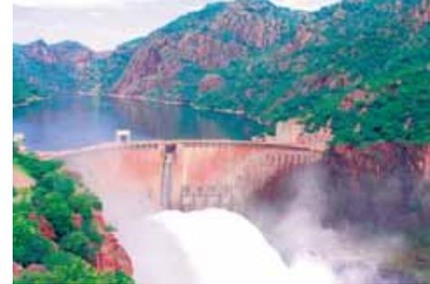
**The dam is 23m thick at its base, 4m at the crown, and has a total discharge capacity of 14,000m<sup>3</sup>/s**
