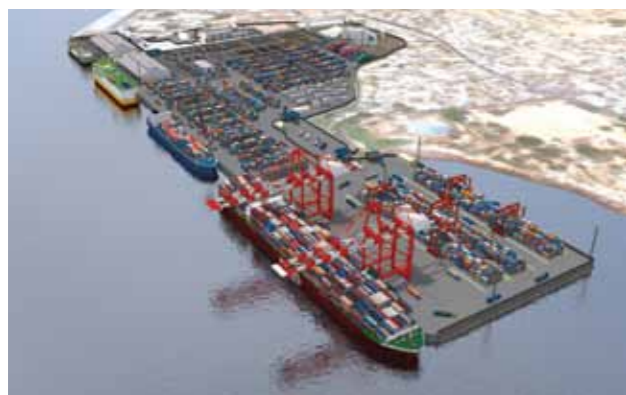
Last October, Bolloré started the $120 million expansion works at the Port of Freetown, one of the biggest investments in Sierra Leone's history
