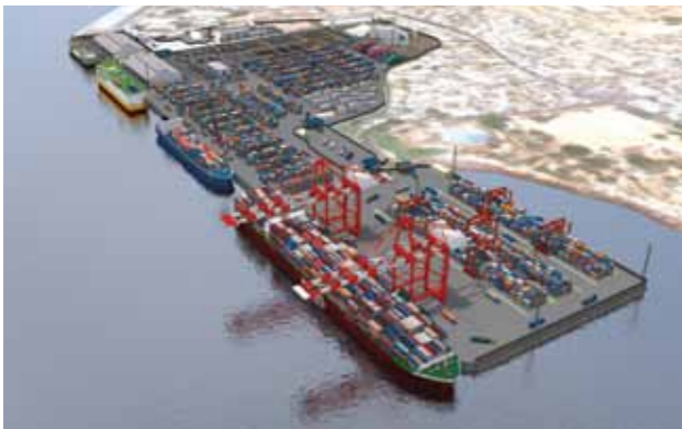
Last October, Bolloré started the $120 million expansion works at the Port of Freetown, one of the biggest investments in Sierra Leone's history
