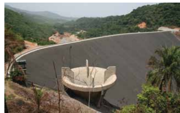
Bumbuna II is the expansion of the 50 MW Bumbuna plant, on the Selu River
